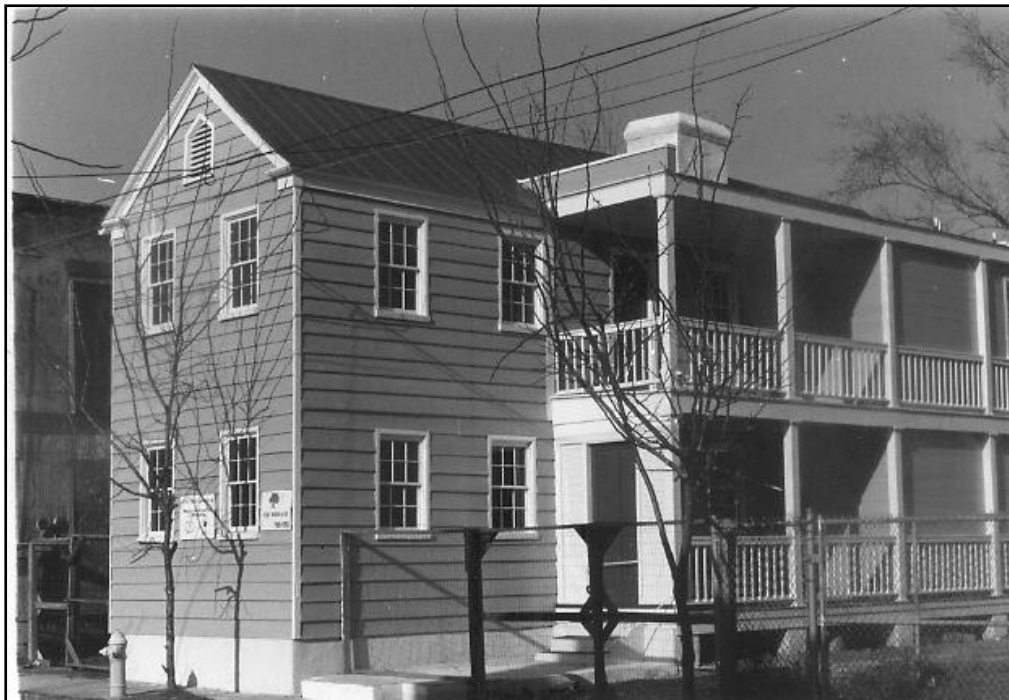
Figure 1: View of the front of 70 Nassau Street after renovation, 1991
