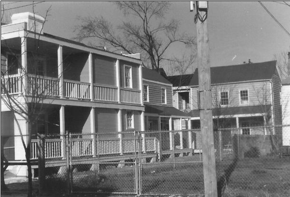
Figure 13: Rear buildings at 70 Nassau Street
